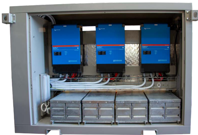
Above: Internal configuration of a custom built 24kVA Energy Pod with MPPT's installed. Please note that these pictures are indicative only & inverter and battery sizes may differ.
